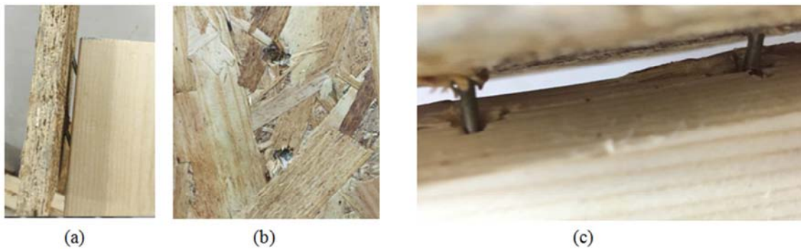
Figure 6. The failure modes of nail joints: (a) nail bent and withdrawn from the studs; (b) nail heads pulled off the panels; (c) split off along the stud grain by nails.
